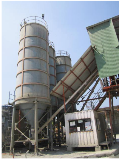
Figure 1 Steel Silo at RMC, Ernakulam
