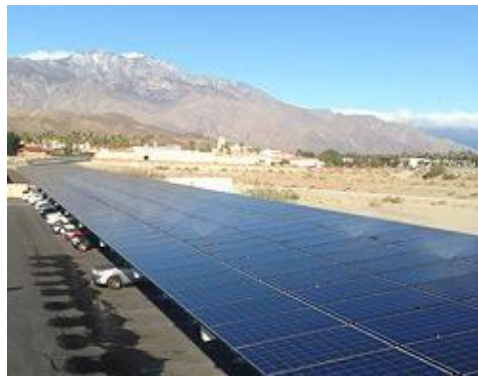
Fig 1.1: Row of solar panel
